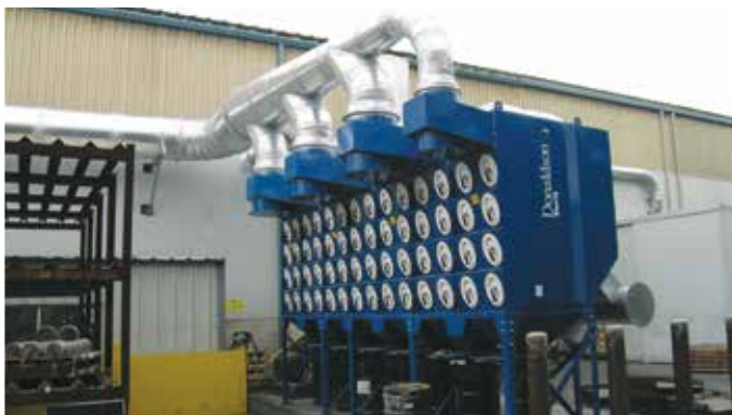
DFO 4-112 on Titanium Grinding
